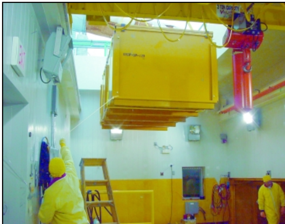
A mobile crane was used to lift out the waste containers from the enclosure for placement in storage and eventual disposal.
