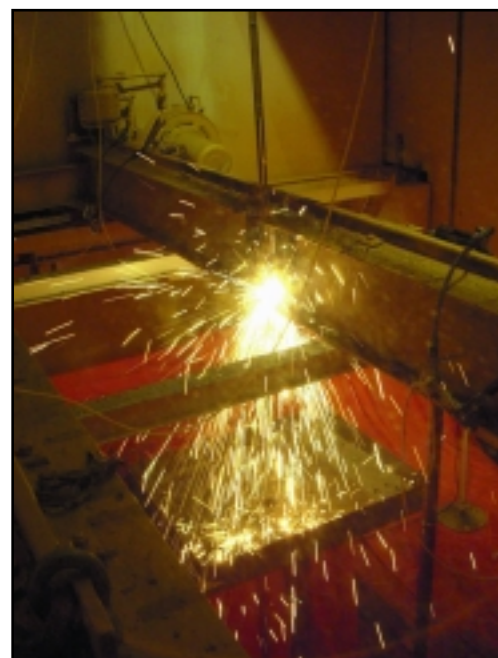
The oxy gasoline torch at work on the failed cranes.
